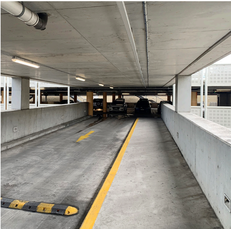
Locally made Olevon Plus installed at a Westfield car park
